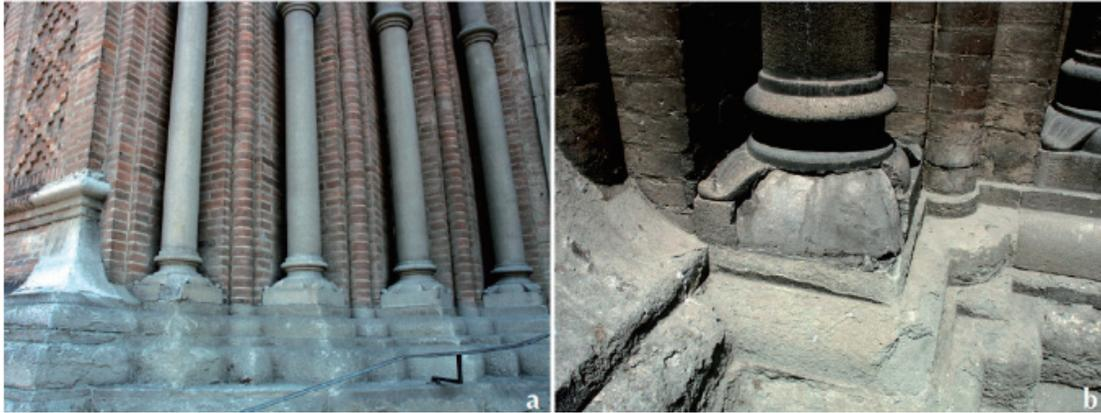
Figure 6. a) Precast concrete columns on a weak sandstone base in the Sacro Cuore Church in Bologna, Italy; b) detail of a column where the external cement-based mortar layer is detached from the concrete core
