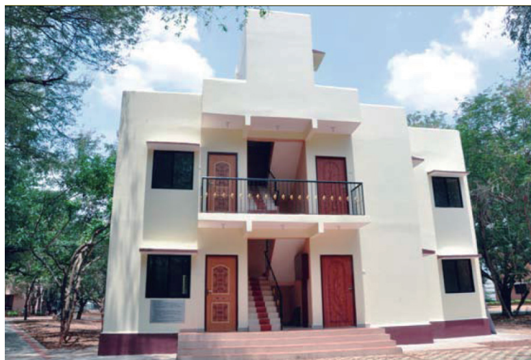
Figure 16. Staff housing quarters with the help of GFRG panels at IIT Madras, India
