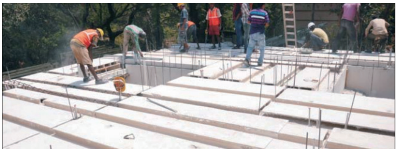
Figure 4. GFRG Roof panels and the reinforcement being laid in micro-beams
