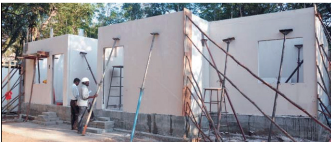
Figure 2. Erection of Wall Panels with Temporary Supports
