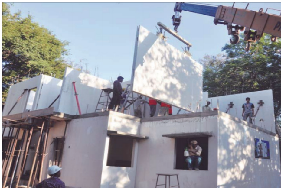
Figure 6. Erection of Panels at First Floor
