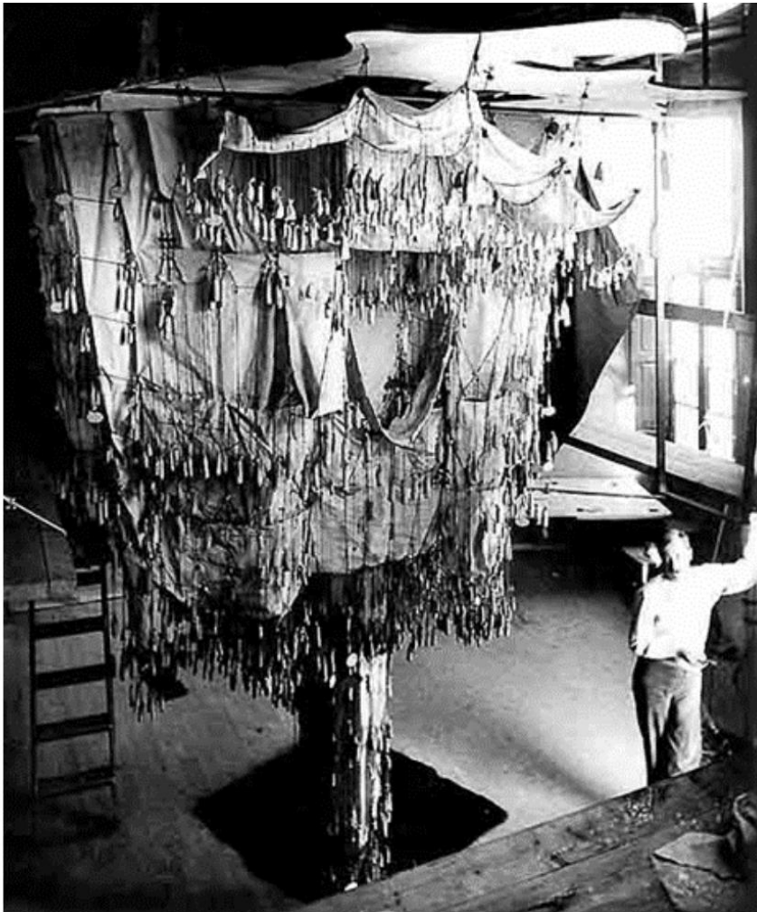
Figure 1. Rope pendant model, small sandbag, and silk paper. Antoni Gaudí. Source: Puig Boada, 1976.
