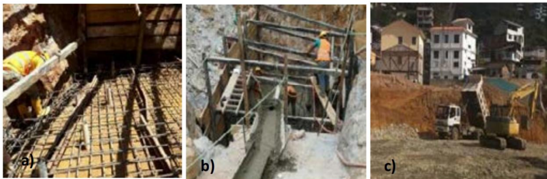
Figure 4. a) Backfill + drains + perimeter beam + iron reinforcement. b) Casting of slab. c) Backfill with compacted material Sub-Base class 3.
