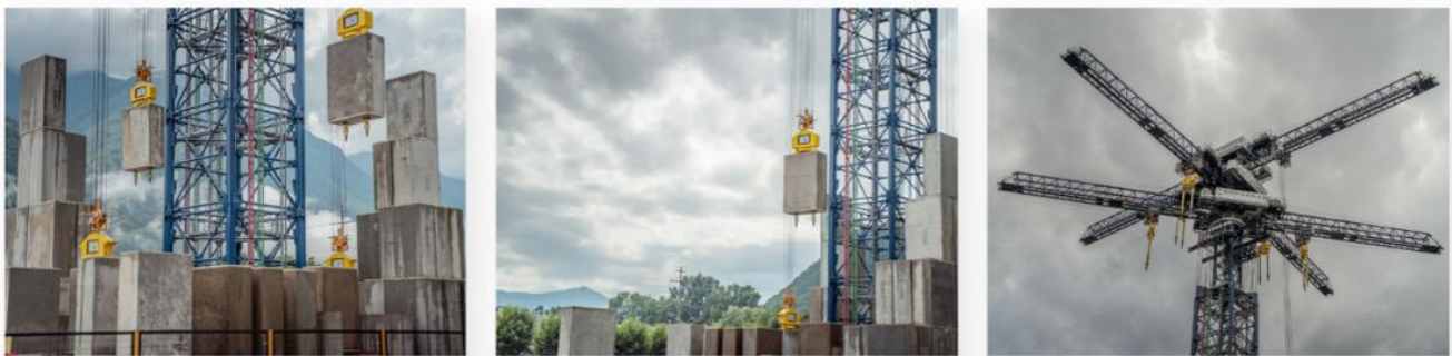
Figure 1. Vault energy gravity pile. Proof of concept executed in Switzerland (Energy Vault, 2022).
