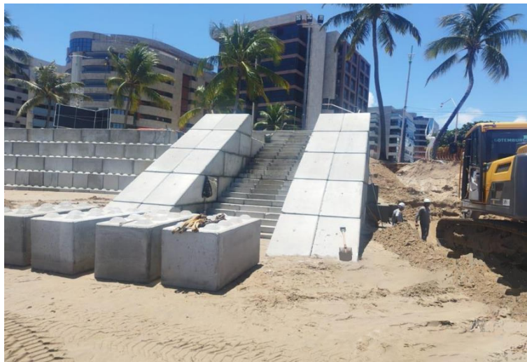
Figure 2. Interlocking precast concrete blocks. Source: the authors
