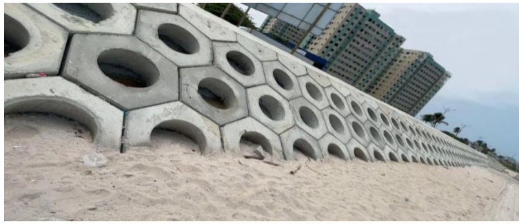
Figure 1. Precast concrete hexagonal rings. Source: the authors
