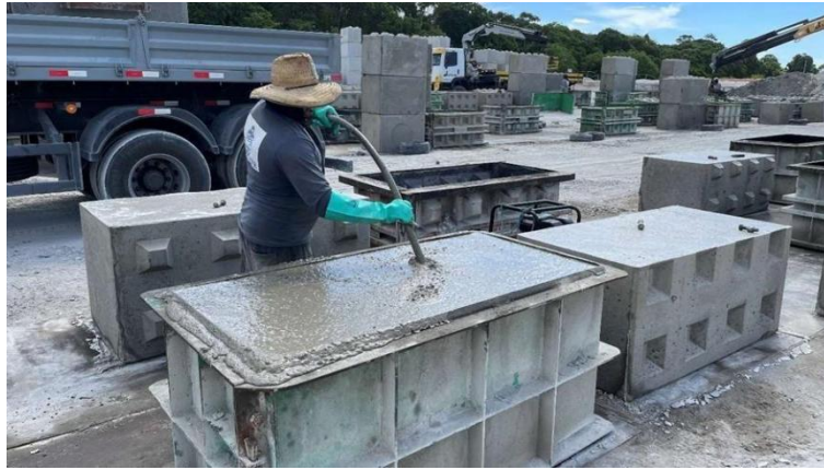
Figure 7. Vibration of the concrete poured into the molds. Source: the authors
