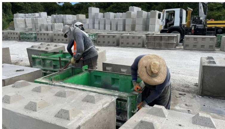
Figure 6. Assembly of metal molds for manufacturing solid blocks. Source: the authors
