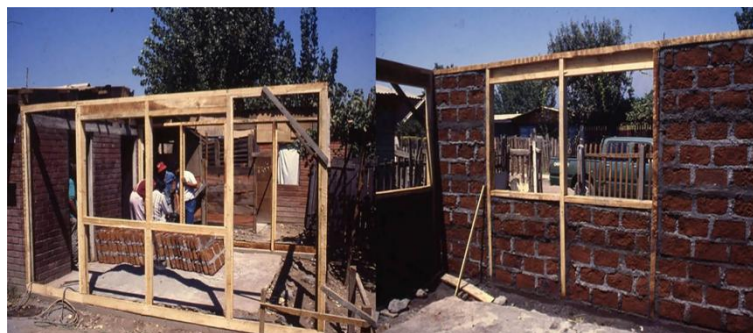
Figure 6. LAD-MA wall assembly process
