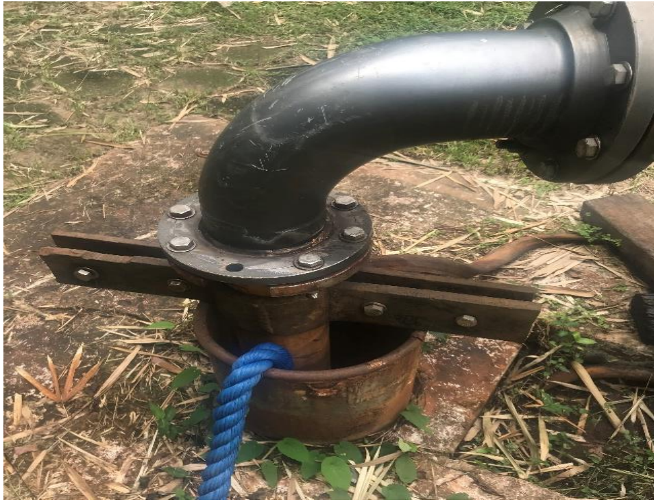
Figure 8. Partial view of the mouth of the artesian well.Source: Authors (2023)
