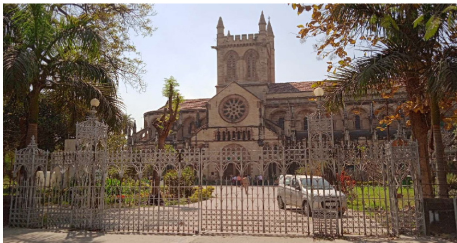
Figure 3. All Saint Cathedral at Allahabad, India.
