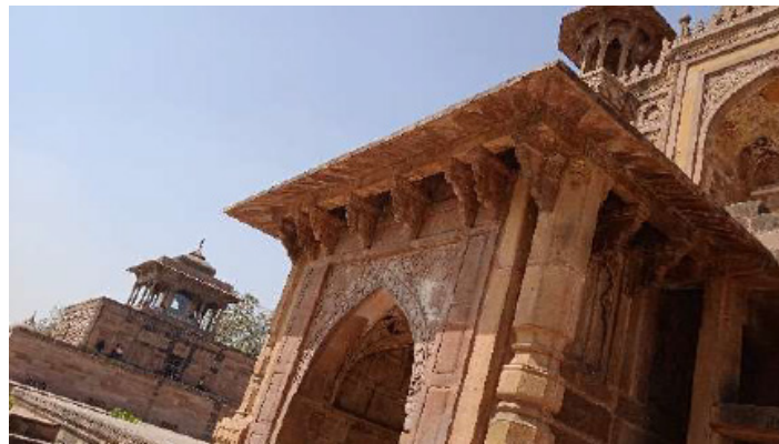
Figure 16. The corbels above the arch.
