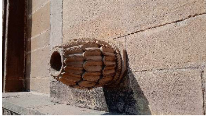
Figure 15. Details of a carved spout for water drainage.
