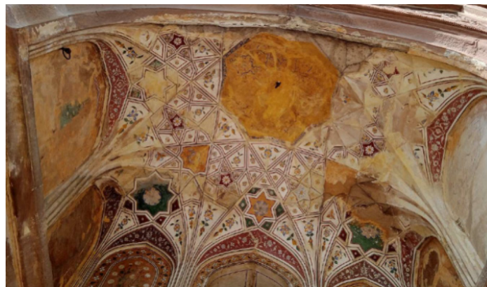
Figure 17. Pendentives and stucco work in the archway.
