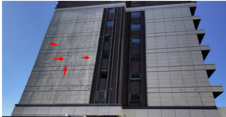
Figure 2. Plate cracks
