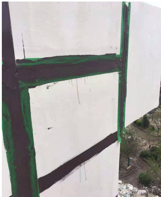
Figure 9. Construction drawing of secondary glue joint
