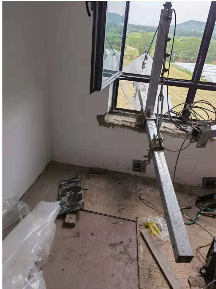
Figure 12. Implementation diagram of the non-counterweight hanging basket at the longitudinal wall
