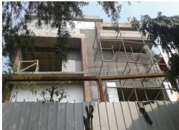
Figure 16. The insulated EPS tiles cladding on external walls
