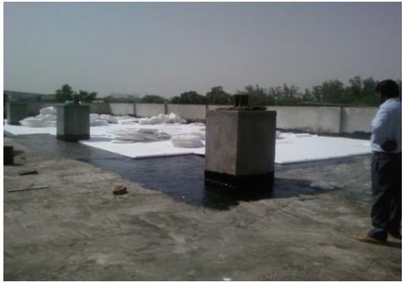
Figure 12. The insulated EPS sheets are laid on the terrace over a bituminous coat
