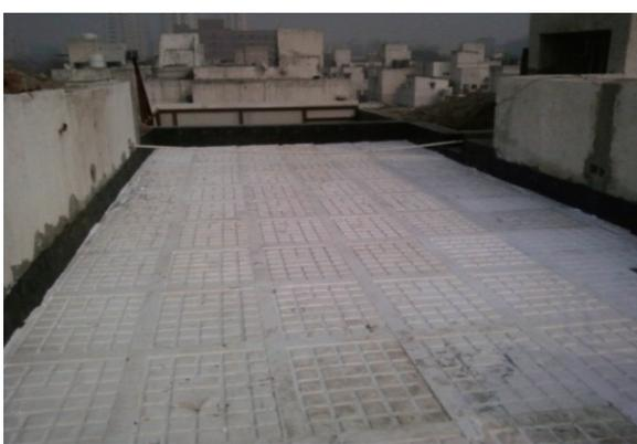
Figure 14. The final finished roof surface with insulated EPS tiles
