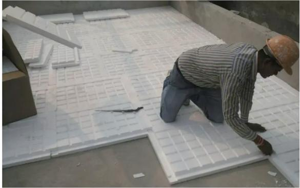
Figure 13. The interlocking insulated EPS sheets laid on the terrace
