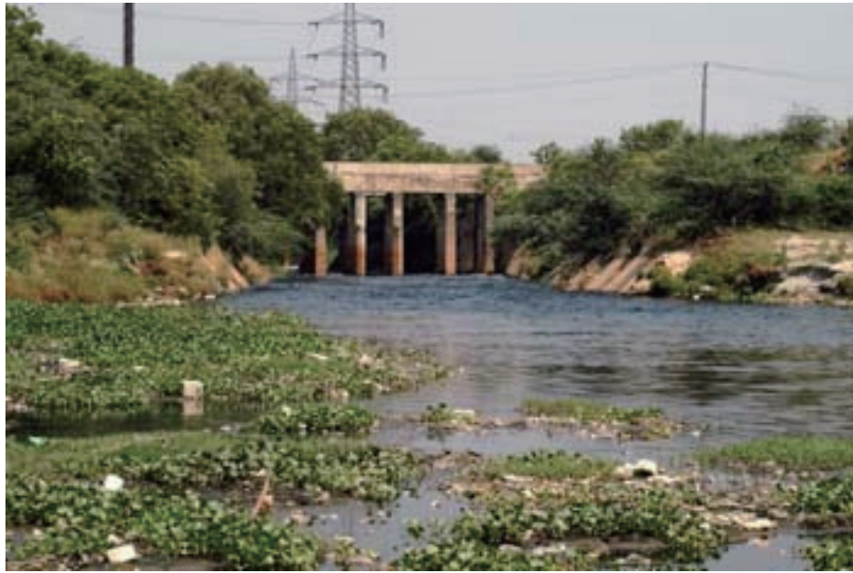
Figure 14. View of Nazafgarh drain
