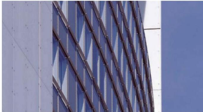
Figure 11. Detail of 125mm ventilation slot with aerofoil strip protruding top and bottom
