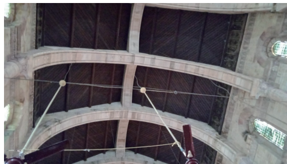
Figure 28. Timber Ceiling over ribbed arches in the Nave
