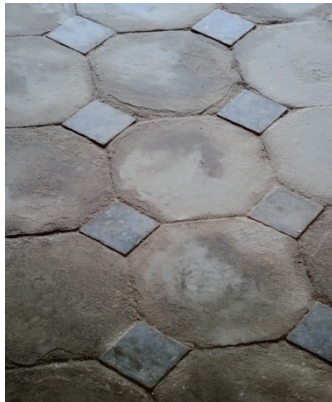
Figure 26. Stone tiles flooring in the Aisle
