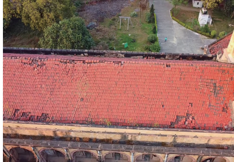
Figure 30. The Terracotta Tiles of the inclined roof on the nave
