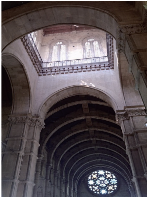
Figure 18. Series of pointed arch on nave
