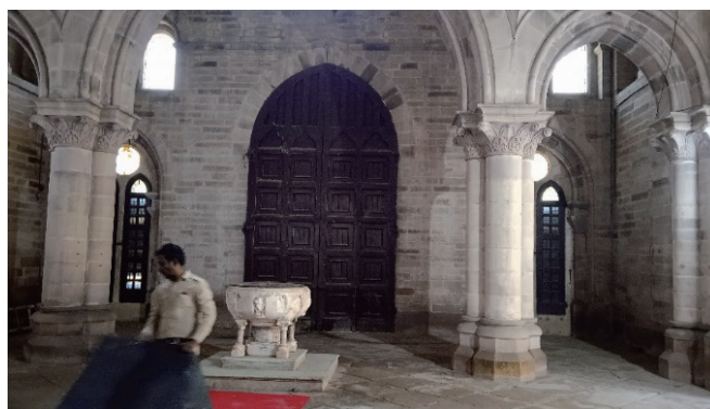
Figure 22. Pointed arch rest on decorated colonnade
