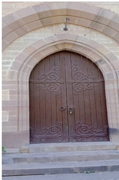
Figure 17. Pointed arch on entrance gate of nave
