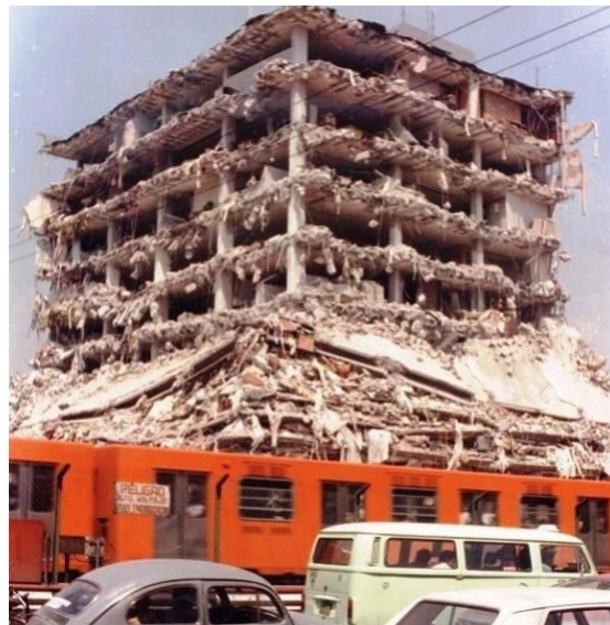
Figure 1: Mexico Earthquake Site
