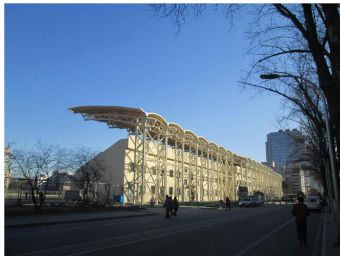
Figure 1. Stadium grandstand canopy
