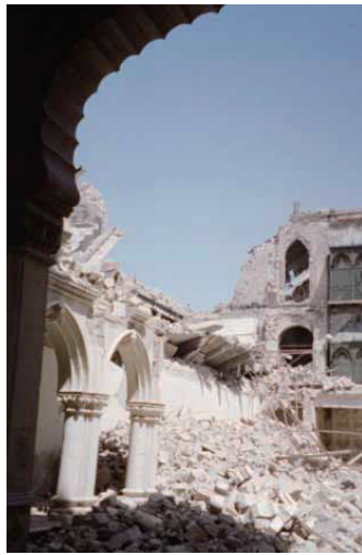
Figure 1. The extensively damaged old palace of Dabargadh
