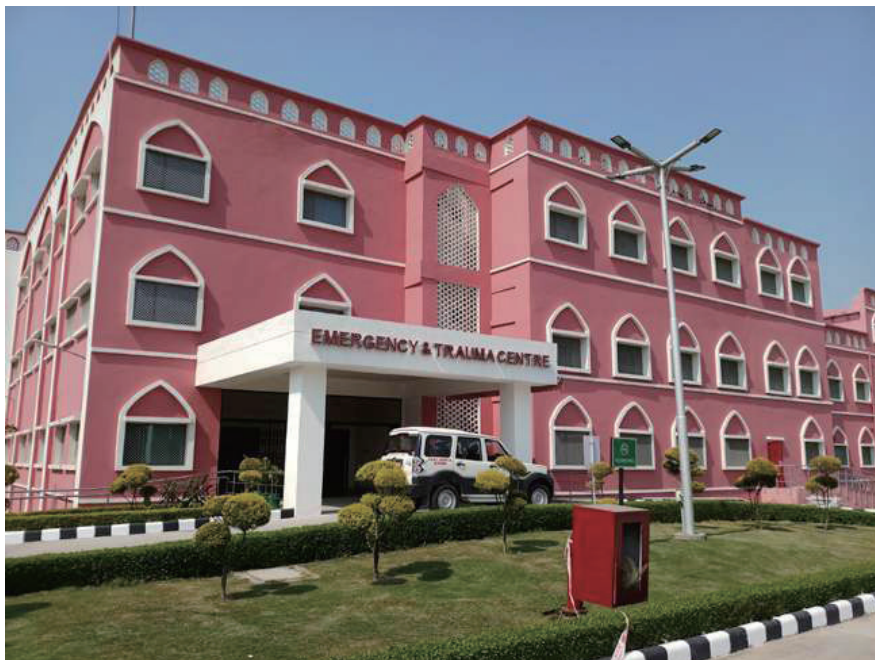
Figure 3. View of the Emergency and Trauma Centre
