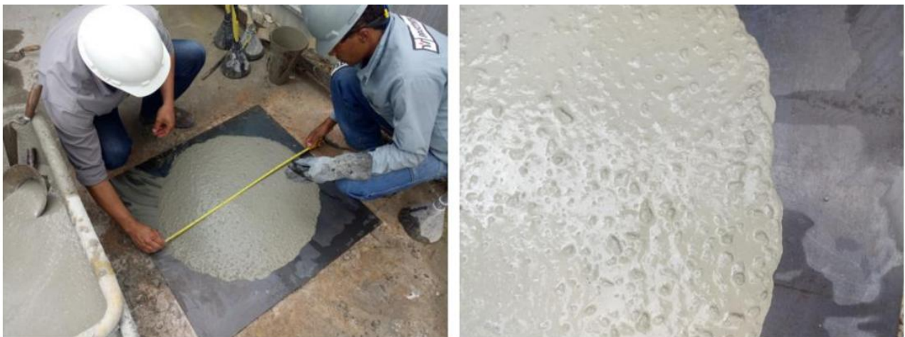
Figure 15. Appearance of self compacting concrete used to reinforce structural formwork.
