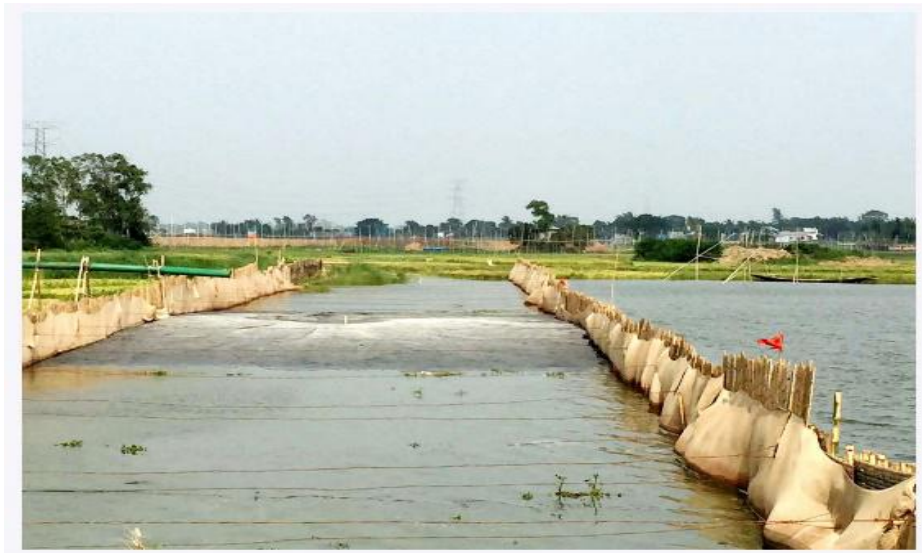
Figure 8. Bamboo structure and sand fill
