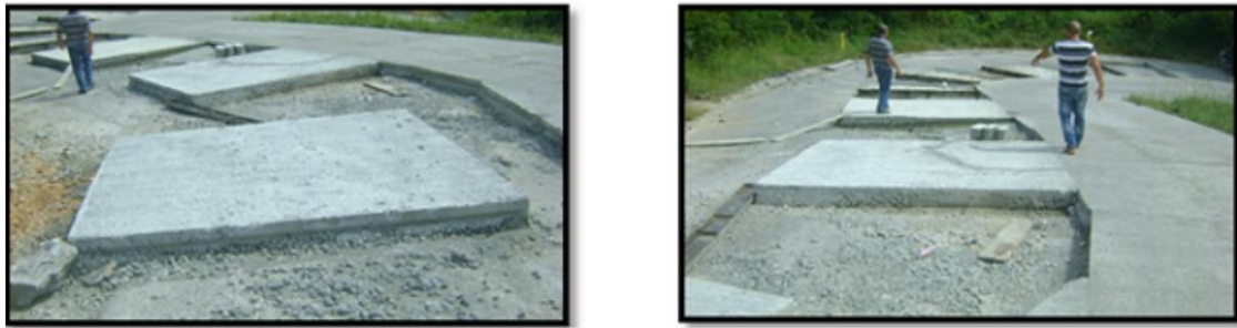
Figure 1. Casting alternating sections on the track.
