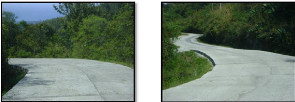
Figure 3. Sections of the rehabilitated road.
