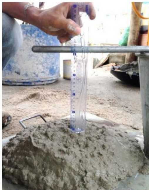
Figure 2. Concrete with slump of around 20 cm. (Source: Author's personal archive)
