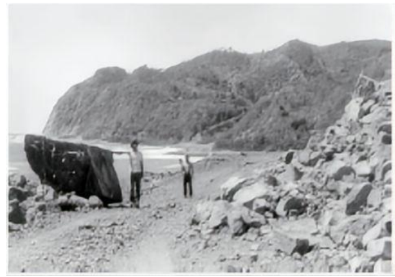
b) Landslide that compromises the road network.
