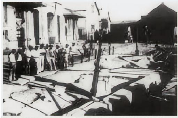
a) Damage caused in the La Alameda area.
