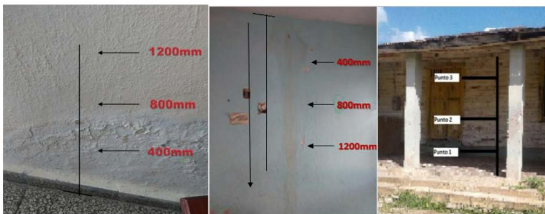
Figure 4. Representation of the points in the measurement zones applied to the 4 typologies. (Authors)
