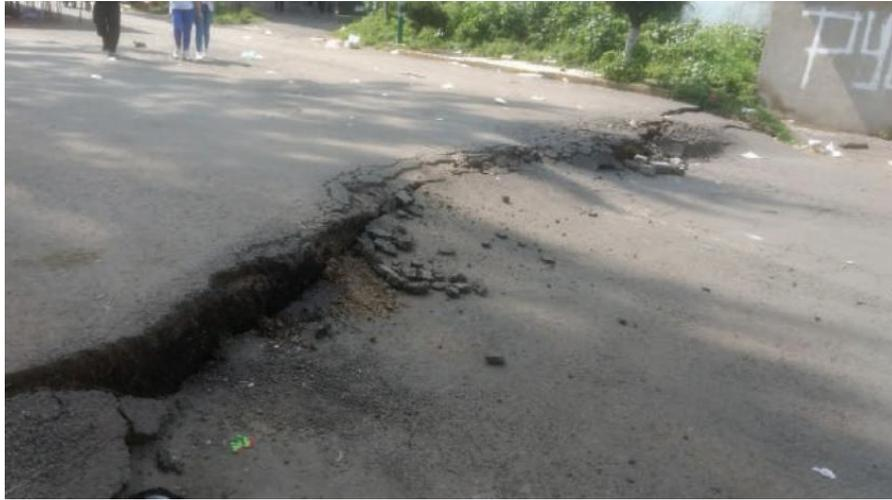
**Figure 1.** Crack with step on a road in Mexico City.
