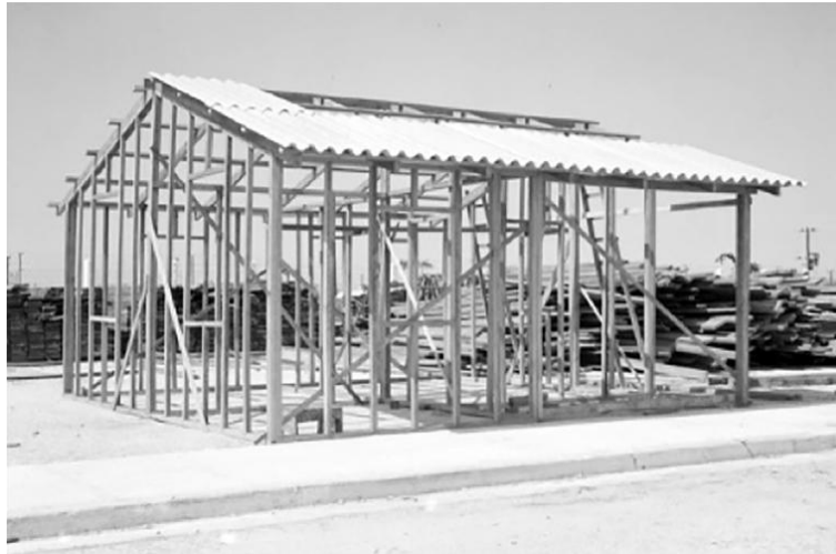
Figure 9. Wooden frame, inspired by Max Borges' prefabricated structures, used in the construction of houses for victims of the fire in Playa Cajío, south of Havana, 1950–1951. Source: Ministry of Public Works Collection, processed and collated by Lic. Juan de las Cuevas Toraya.
