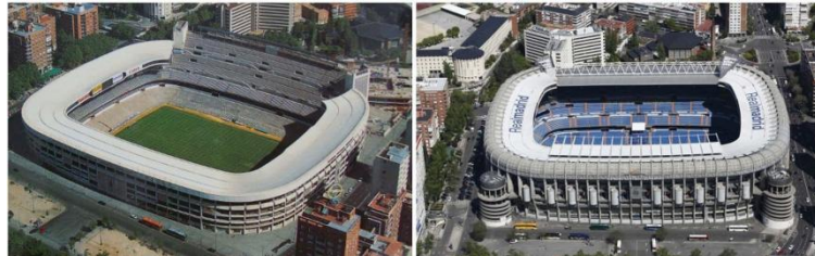
Figure 2. Appearance of the stadium after the 1982 (i) and 1994 (d) renovations
