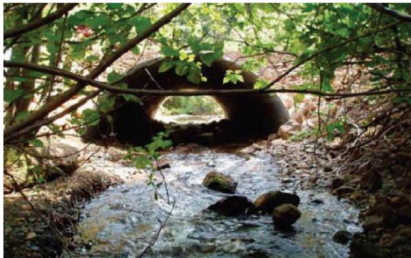
Figure 3. Fully installed open-bottom culvert (adapted from USFS, 2008)
