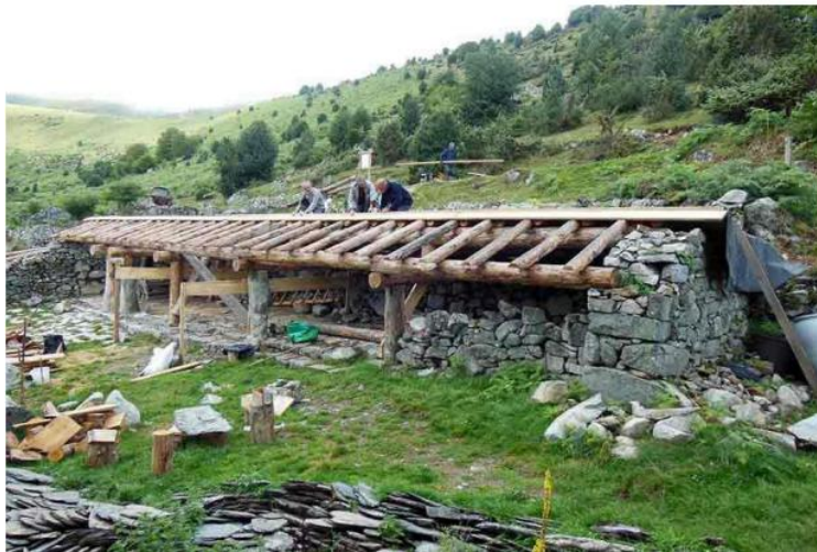
Figure 10. Campan (Hautes-Pyrénées), restoration of the stable © Association Pierre des Esclozes
